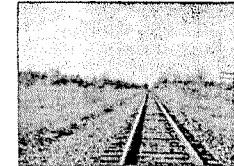
VEN '13' LOOKING NW DOWN CORRAL, S.E.
