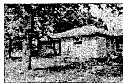
VEN '9' LOOKING NW AT EXISTING BUILDING
