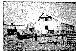
VEN '5' LOOKING SE AT EXISTING BARN
